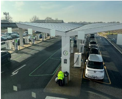
Figure 23: A line of private EVs charge on 90kW (capable) DCFCs at a Gridserve Forecourt, under a Solar PV canopy. A maintenance worker empties trash.
