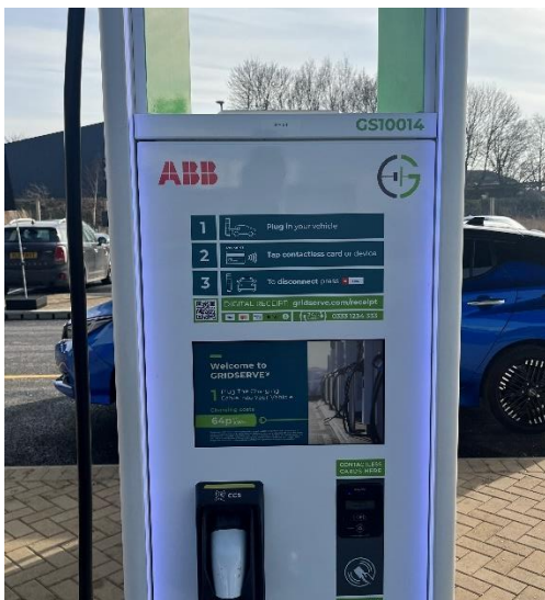
Figure 16: A 350kW capable DCFC made by ABB at a Gridserve forecourt. Plug type is CCS2, payment can be either contactless bank/credit card or a membership app/card.
