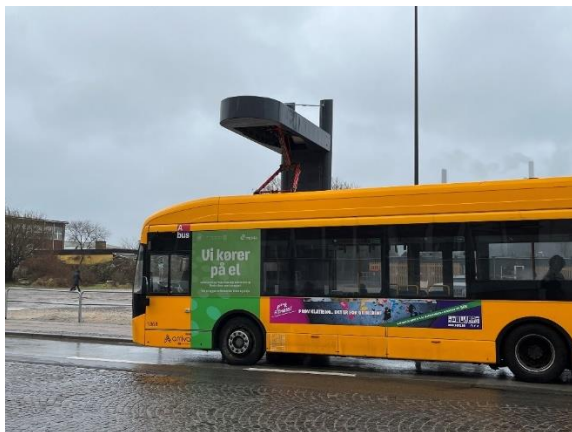
Figure 8: City Bus charging on a 450kW Pantograph in Copenhagen, Denmark
