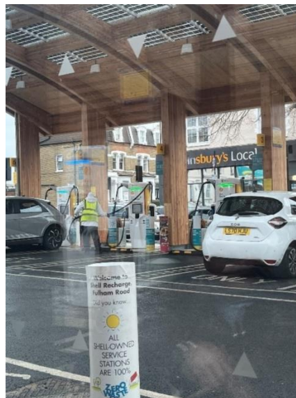
Figure 20: A technician maintains DCFCs at a Shell Forecourt.
