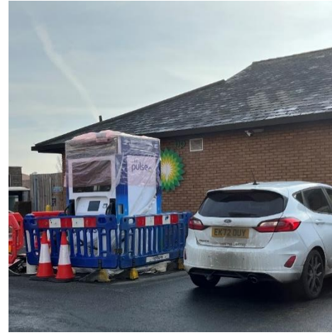
Figure 4: A bp pulse dual DCFC waits to be installed at an already crowded and power constrained forecourt.
