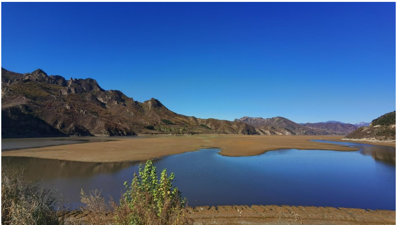
Figure 4: Miaogong Reservoir, which has entirely lost its capacity and function due to serious sediment deposition (photo by Jiaheng Zhao).
