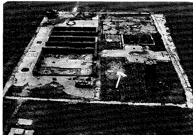
Fig. 2. The Brunel Scab that replaced the old eyesore in 1975; it remained in this unfinished state for a further two years. The picture shows clearly the old foundation-line, which would have to be followed in the new scheme
