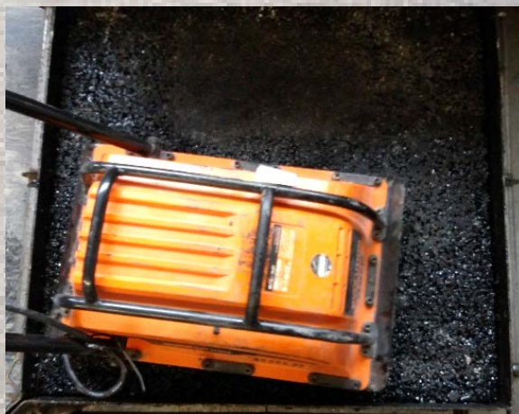
Asphalt fill compacted in pothole
